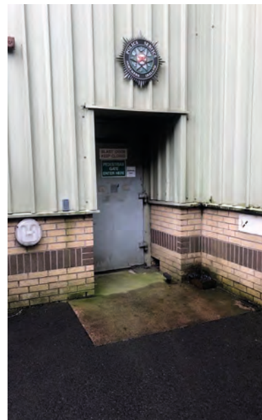
7. Newtownhamilton Station public main building entrance
