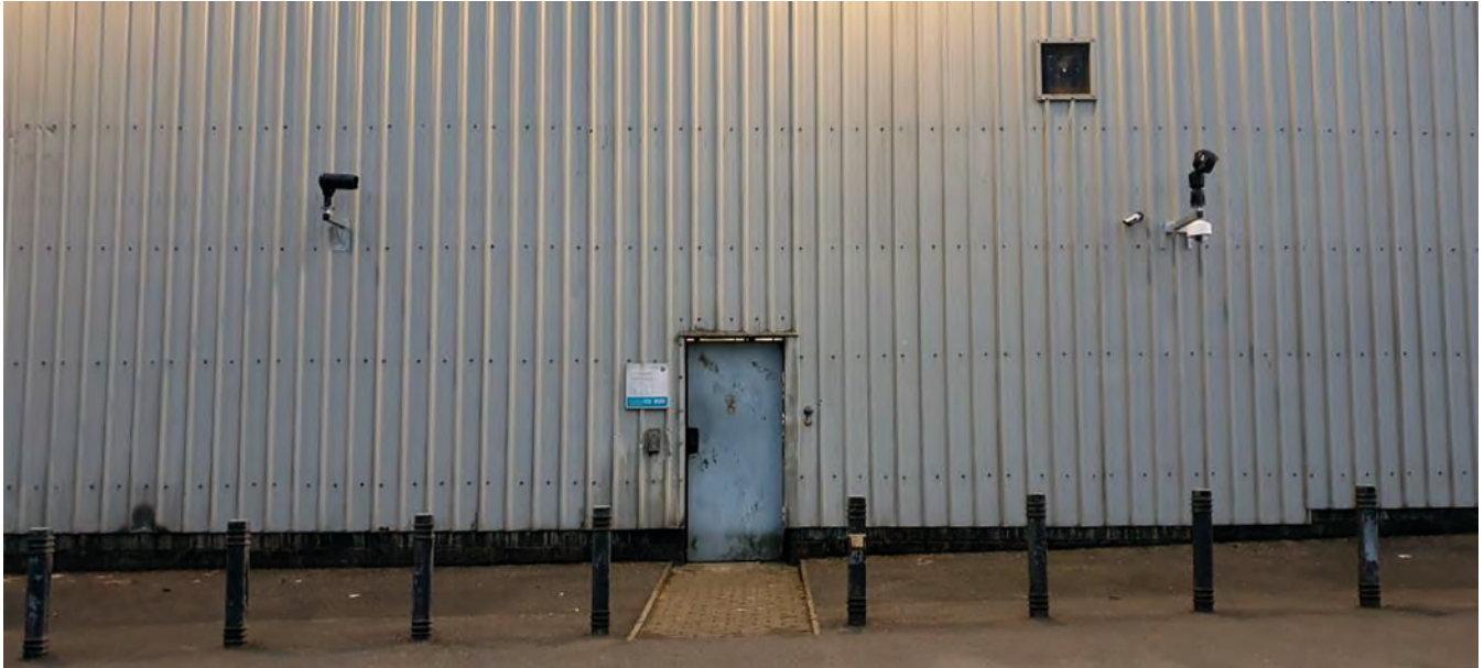
3. Crossmaglen Station front façade – public pedestrian entrance
