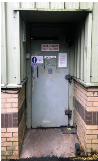
9. Newtownhamilton Station street access view
